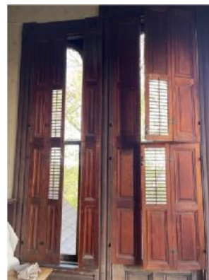
Windows in the tower room are working and sealed. Thank you Mark and Elizabeth.
