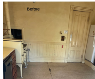
2021 kitchen before new floor and fresh paint
