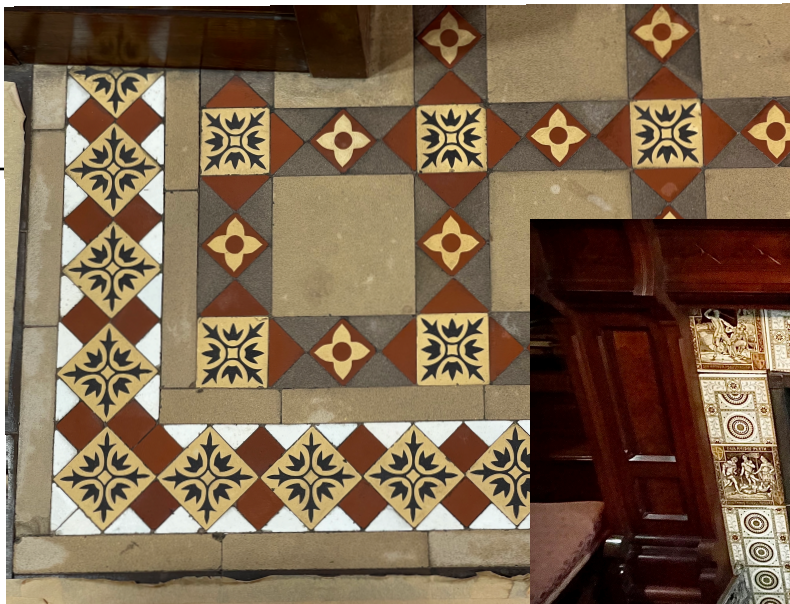
The cleaned and sealed corner tiles.
